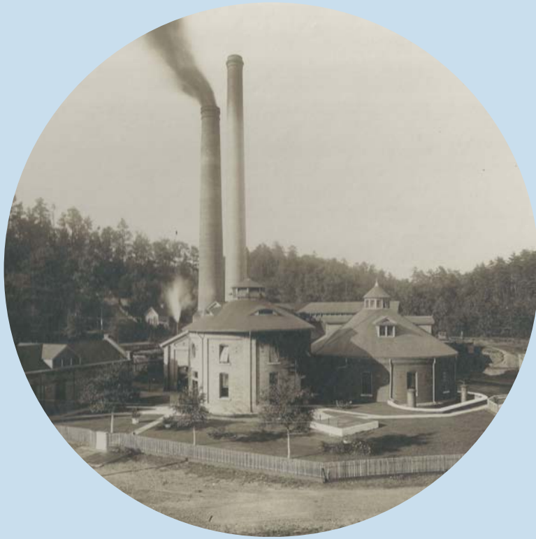
Cahaba Pumping Station
