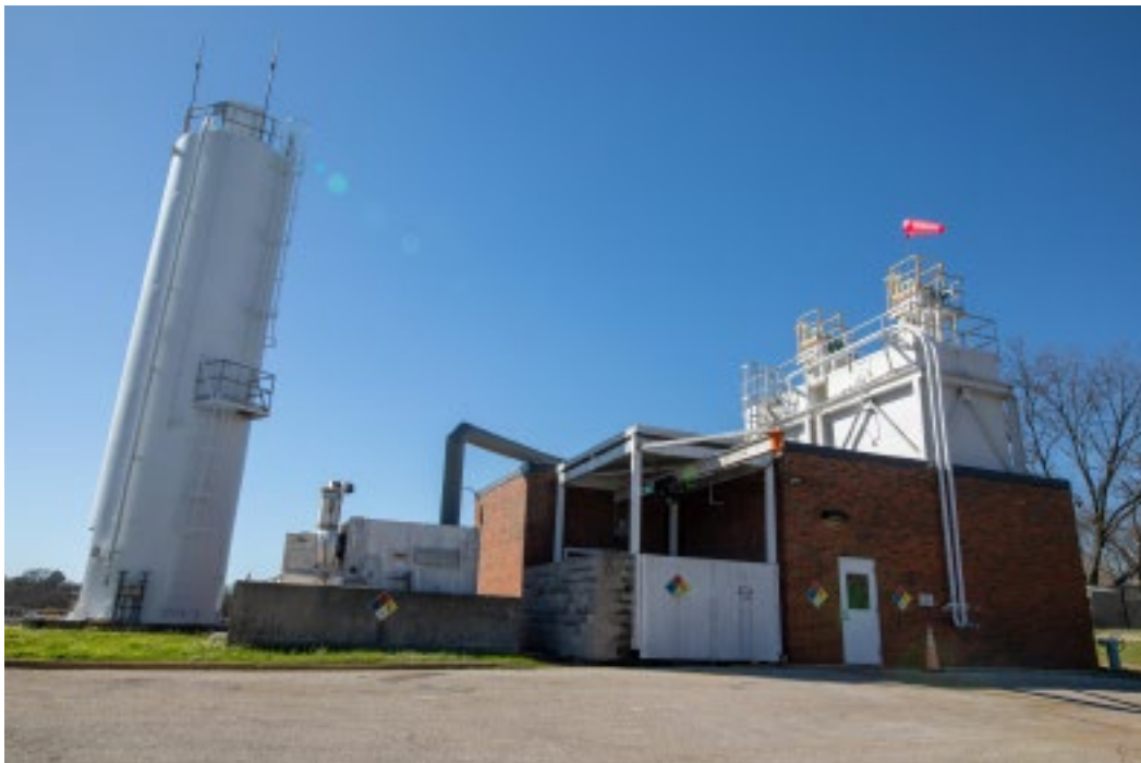
PUTNAM FILTER PLANT
