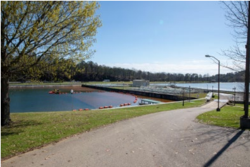
SHADES MOUNTAIN FILTER PLANT
