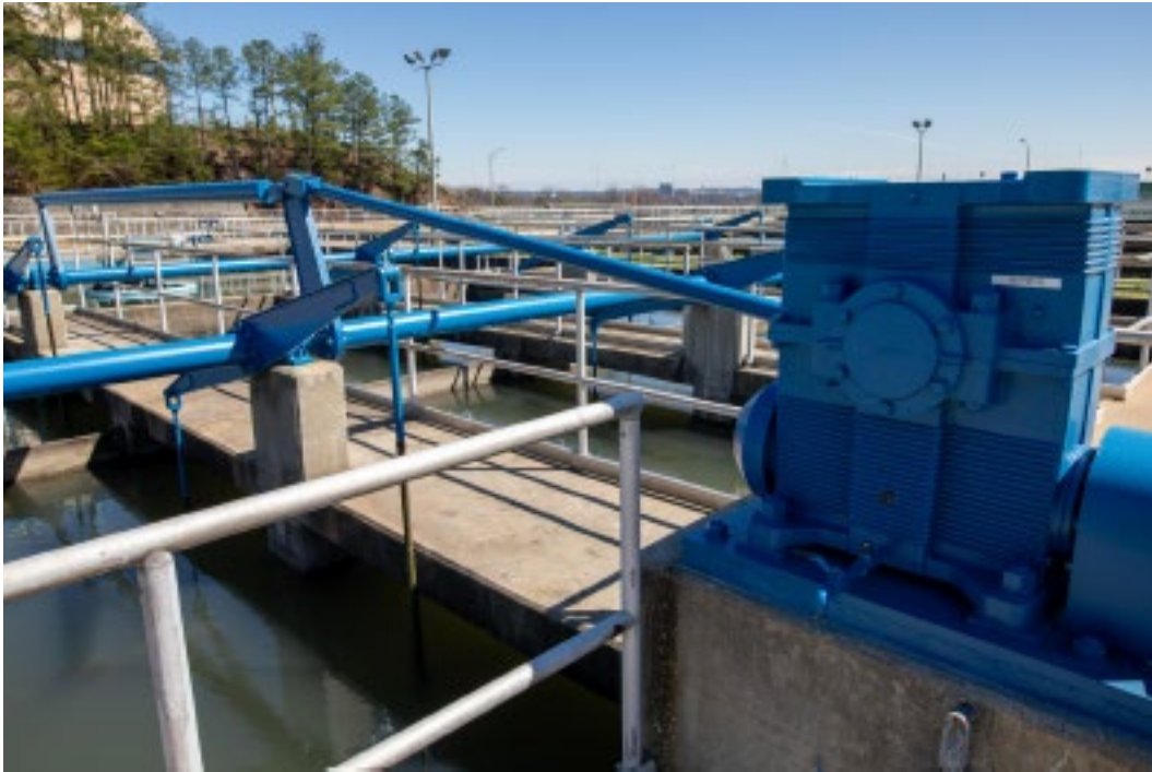
WESTERN FILTER PLANT
