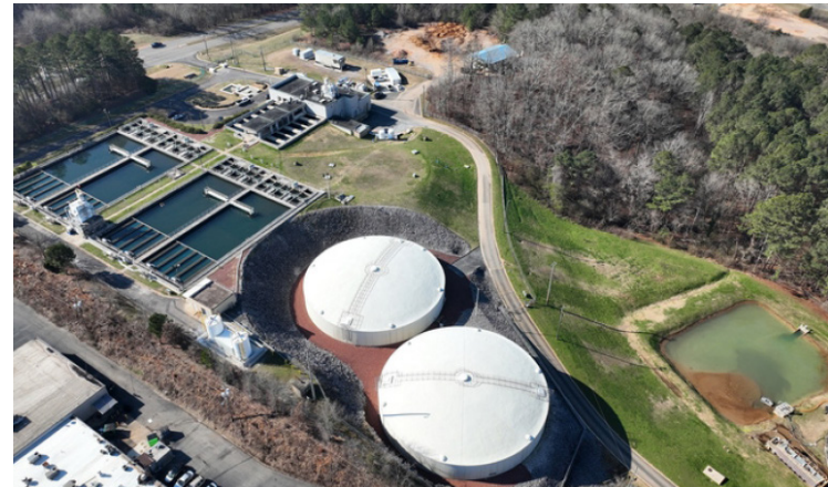
Pictured: Award-Winning Carson Filtration Plant
