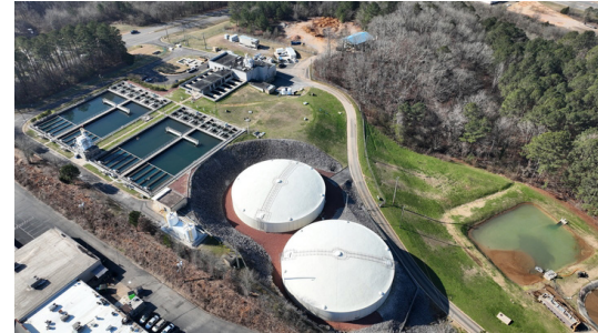
Pictured: Award-Winning Carson Filter Plant
